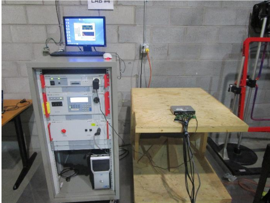
Photo 18: Harmonic Current Emissions – Test Setup
