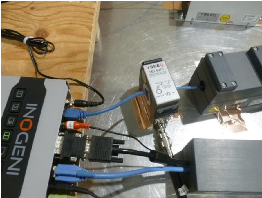
Photo 42 : Conducted Disturbances – Test Setup – EM Clamp – RS-232 (SHARE 2)
